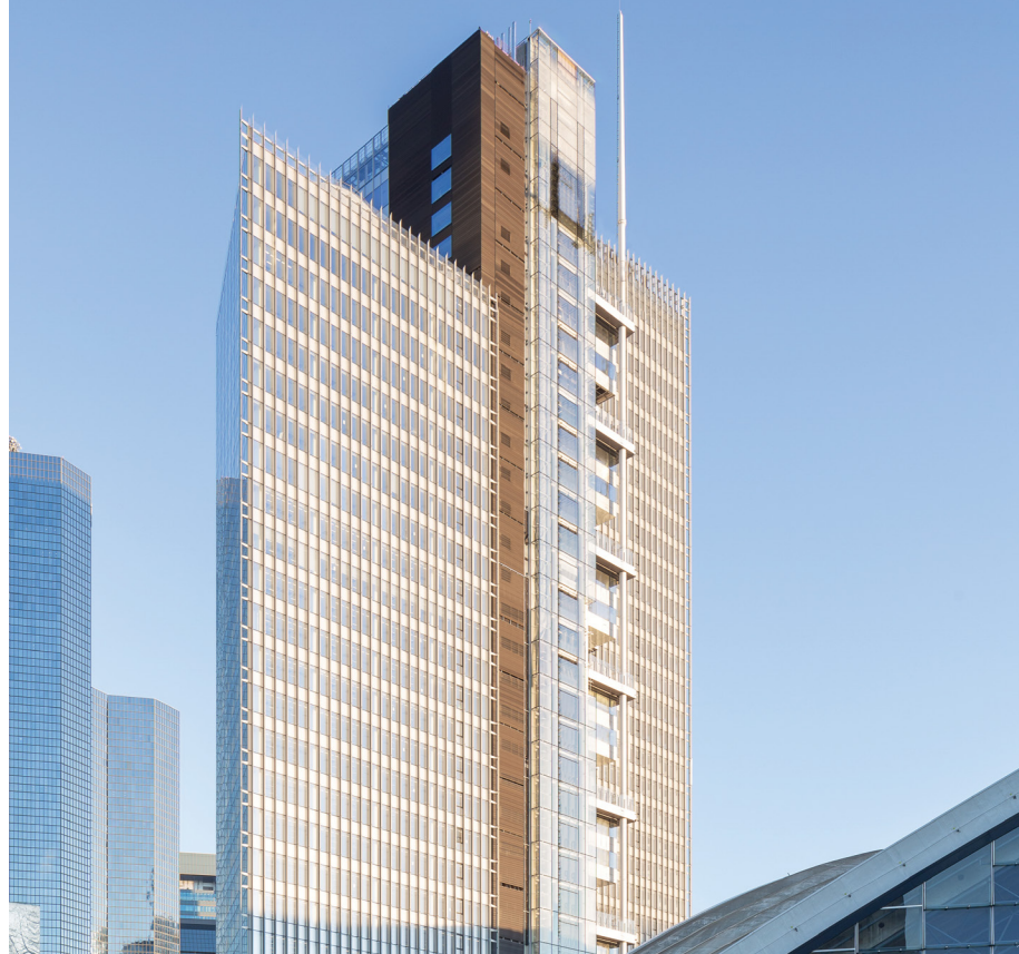
Figure 12. The façade is rendered with printed glass blades that obscure separations and aid solar protection. © Hugo Hebrard
