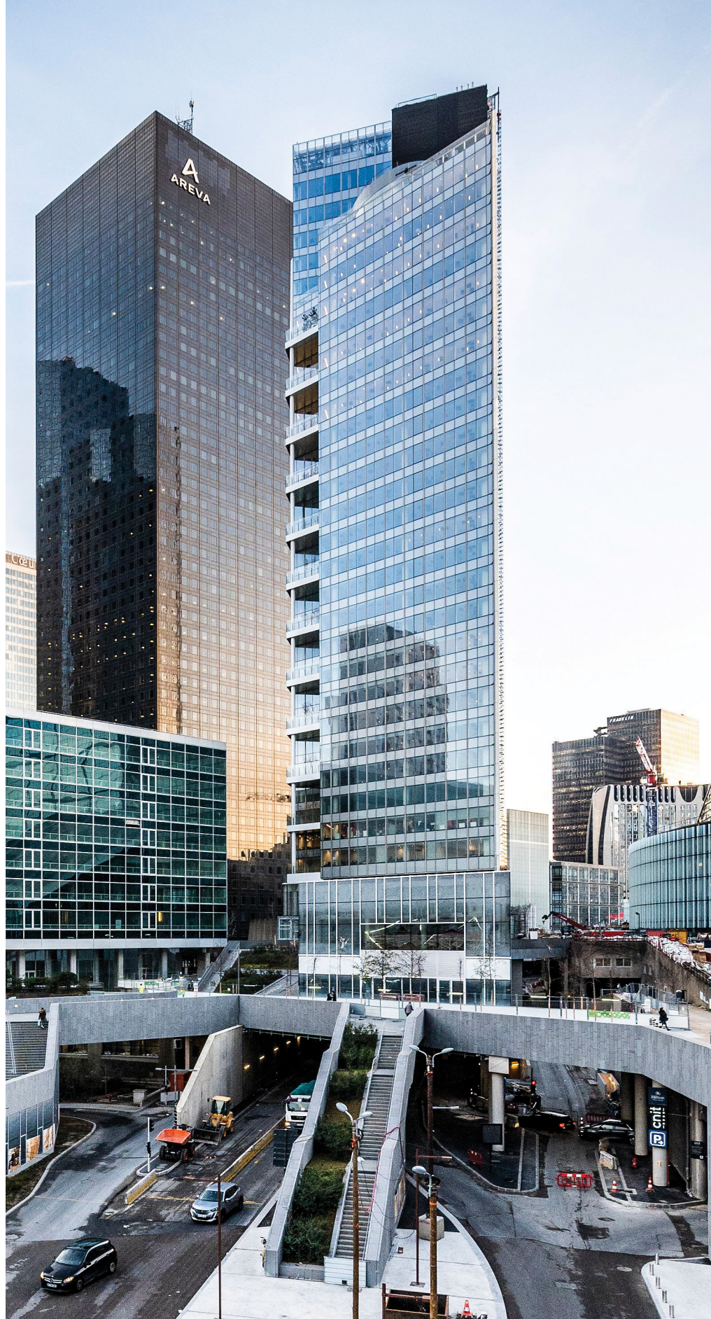
Figure 2. Trinity was a significant site-repair project, resolving grade changes for pedestrians and bridging over an active highway. © Laurent Zylberman
